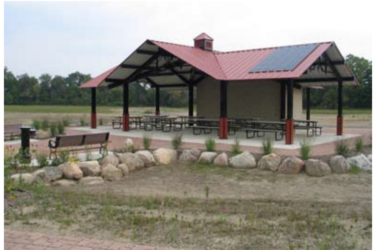
The Pavilion at Riggs Heritage Park features stormwater filtration practices and solar panels. In the same park, the infiltration basin is surrounded by meadow plantings. photo: Van Buren Township
