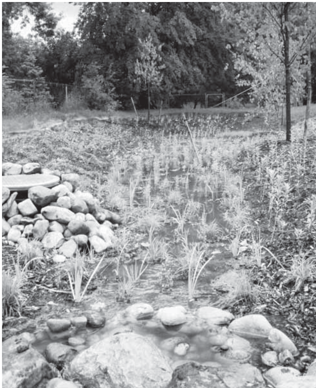
The Briarcliff rain garden is seen here fulfilling its function by trapping rainwater on site so it cannot enter the storm sewer and Millers Creek. photo: HRWC
